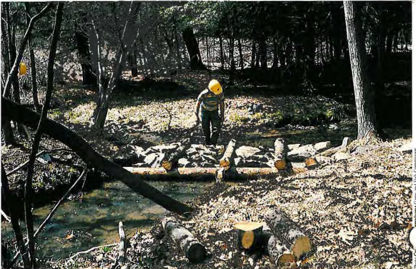
Figure 5. —Channel block - crib.
