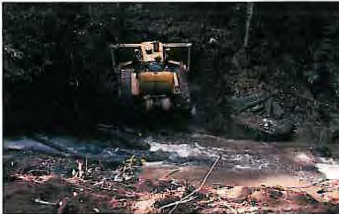
Figure 52.—Bulldozer excavating banks.
