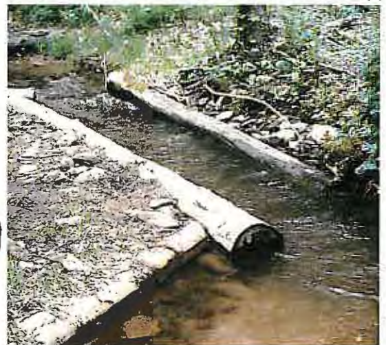
Figure 41.—After channel constrictor installed (18- to 20-inches deep).
