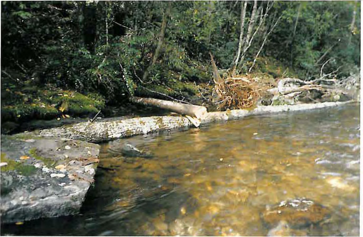
Figure 20. —Log driven into bank and pinned to tree.
