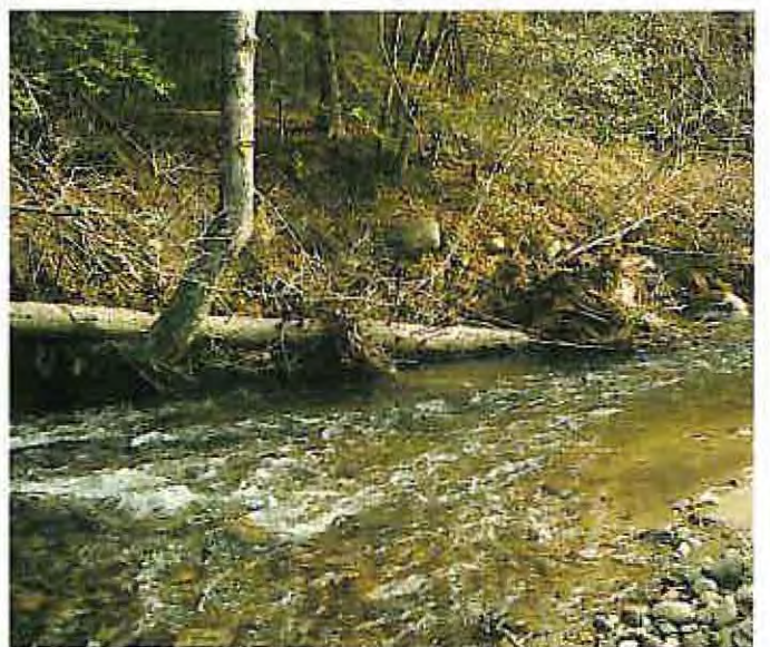
Figure 16. —Rootwad pinned to tree with rebar.
