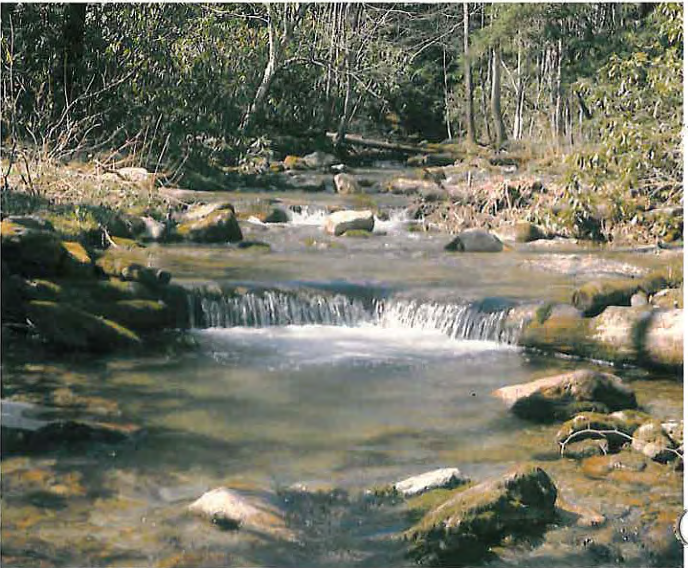
Figure 47.—Wedge dam after 13 years.
