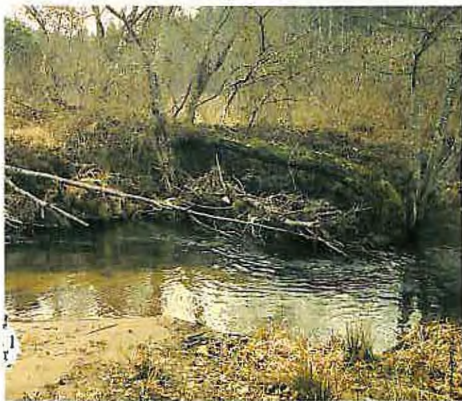
Figure 13. —Rootwads driven into bank.
