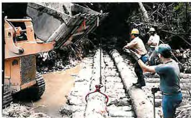
Figure 54.—Placing sill logs.
