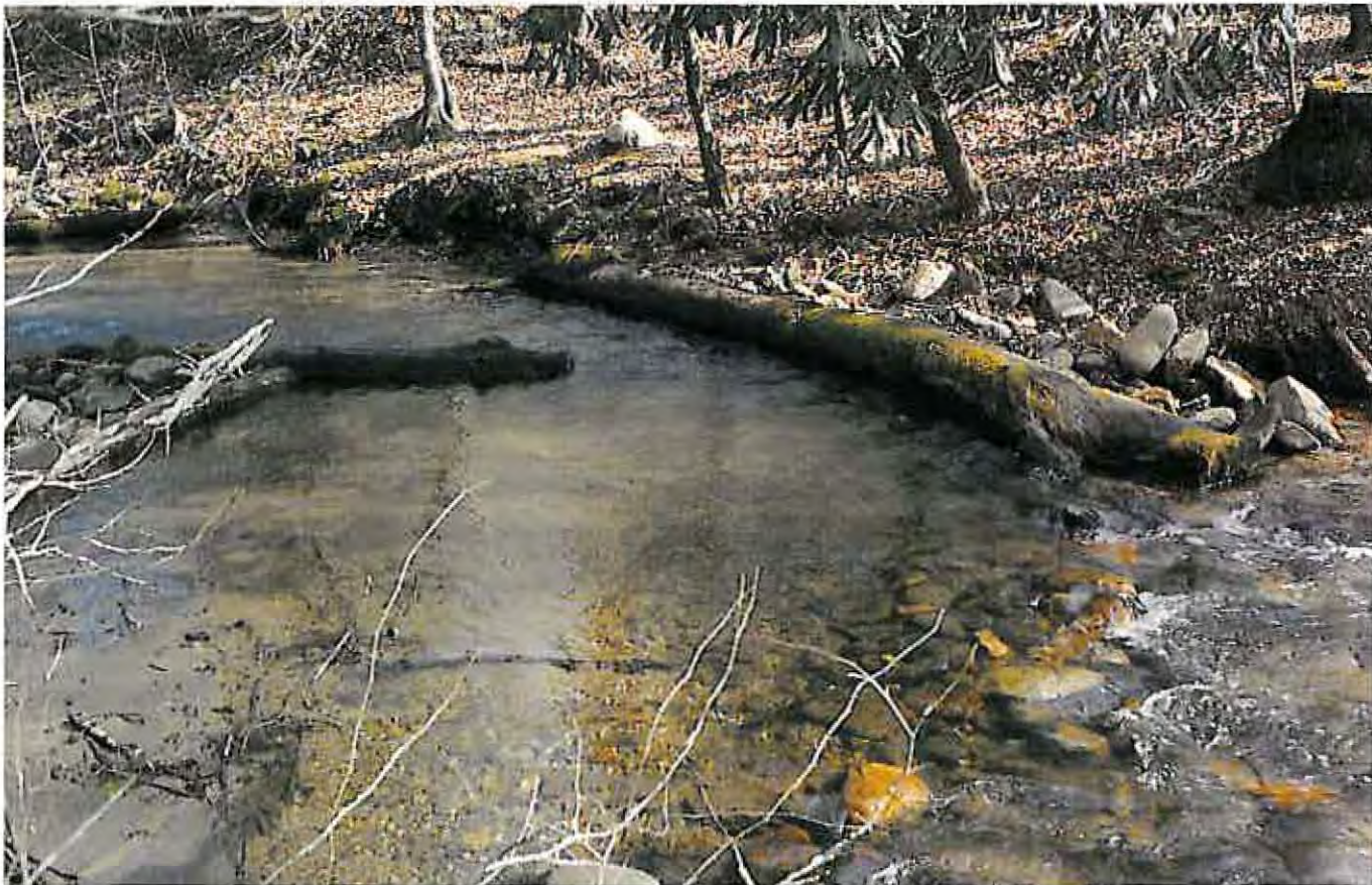
Figure 37. —Deflector and cover log.
