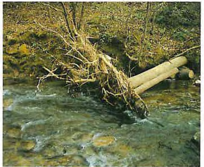
Figure 15. —Single rootwad driven into bank.
