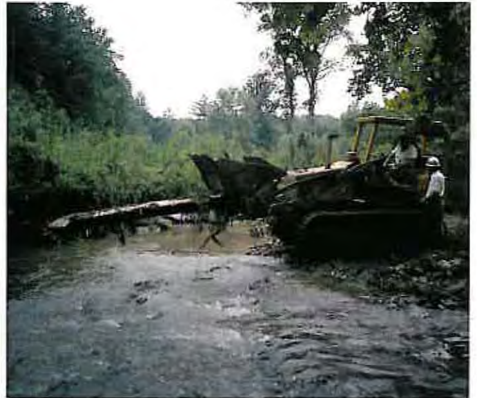
Figure 14. —Driving rootwads.
