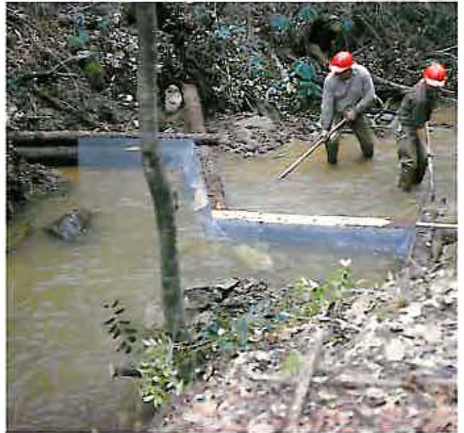
Figure 46.—Wedge dam with wire added.
