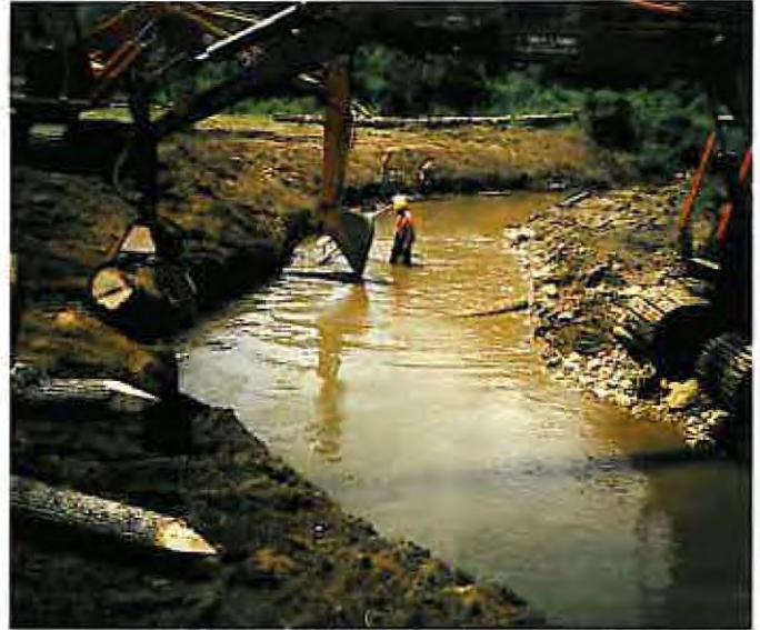
Figure 29. —Driving 12' logs for bank shelf support.
