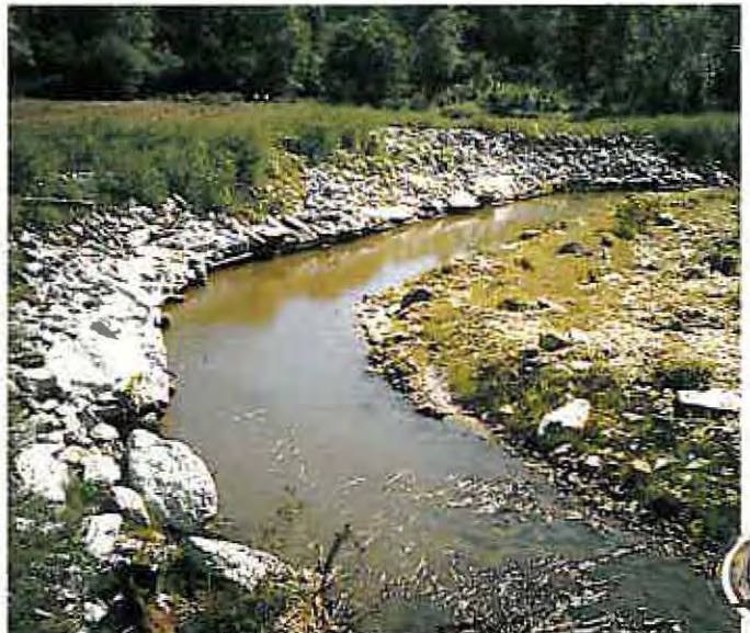
Figure 31. —Shelf with rock added 6 weeks after installation.
