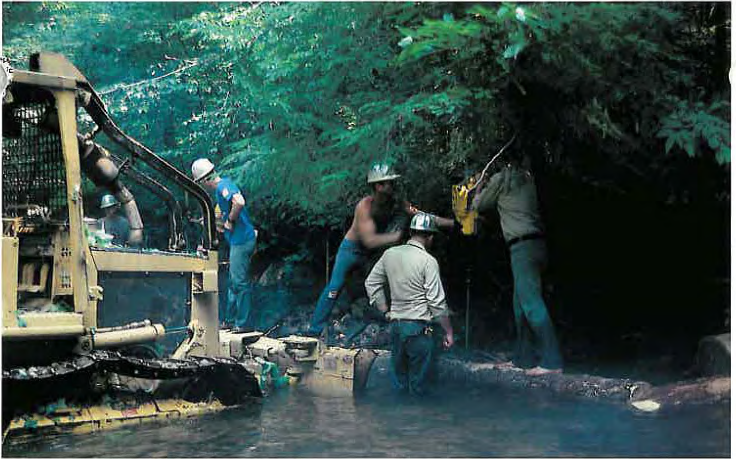
Figure 58. —Driving rebar with Cobra drill.
