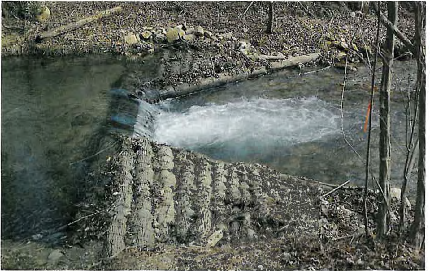
Figure 49. —K dam with log fill in crib.
