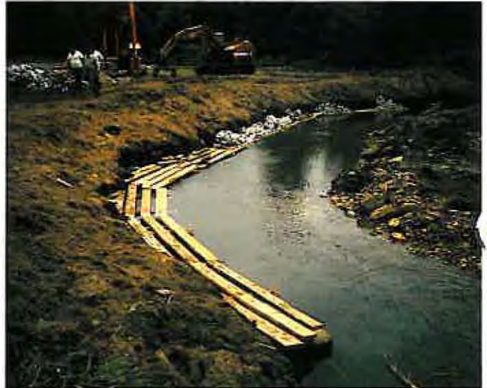
Figure 30. —Adding planks for shelf.
