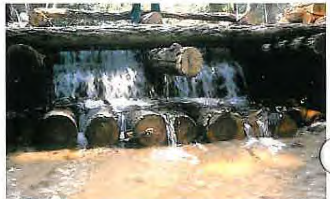
Figure 57.—Water spilling through apron onto log floor.
