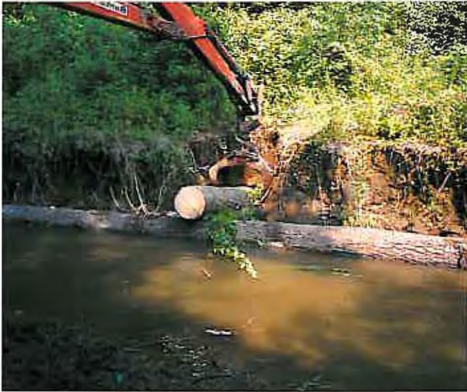
Figure 26. —Placing abutment log on main log.
