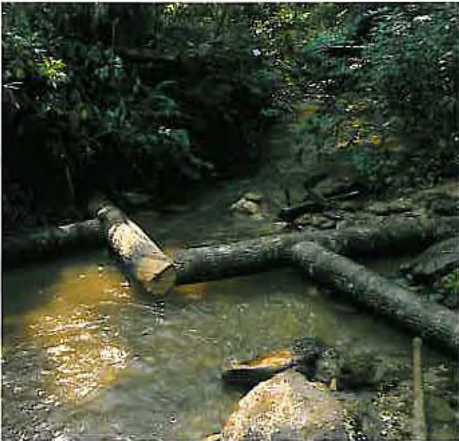
Figure 45.—Wedge dam elevated for pinning.
