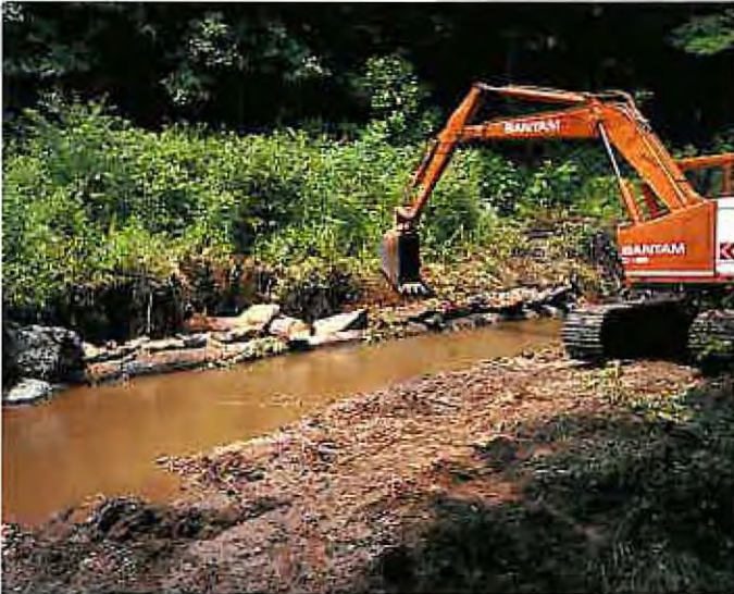
Figure 27. —Adding slab rock and tamping bank.
