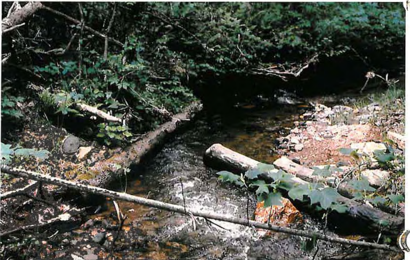
Figure 34.—Deflector and cover log.
