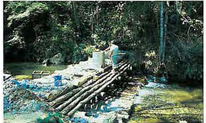
Figure 56.—Completed fish barrier.
