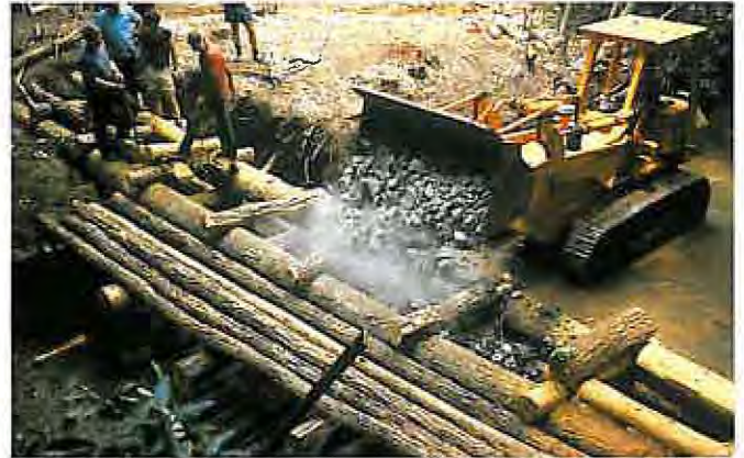
Figure 55.—Filling crib with rock.
