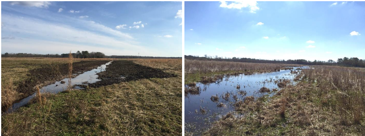
Figures 3a and 3b. Shallow excavation adjacent to a channelized stream creates a wetland that supports emergent vegetation and provides water quality benefits without impeding drainage.
