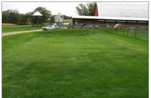
For the wastewater treatment strip to work properly, discharge to and through it must be in the form of sheet flow so that the discharge does not concentrate into channels. Some means, such as a ditch, curb, or gated pipe, is provided to disperse concentrated flow and ensure sheet flow across the width of the treatment strip.
