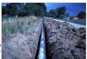
An irrigation pipeline can be made of flexible conduit materials, such as plastic, steel, aluminum, corrugated metal, or ductile iron pipe, or it can be made from rigid conduit, such as concrete or plastic mortar pipe. The pipeline can be installed underground or above ground.
