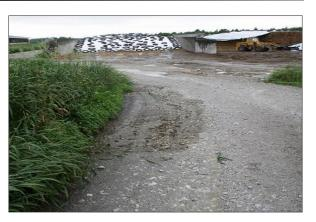
The design of an access road is based on the soils, climate, topography, drainage patterns, and anticipated operating conditions. Surface treatments vary from bare earth to a hardened surface such as asphalt or gravel. Drainage features associated with the practice could include culverts or surface cross drains.
