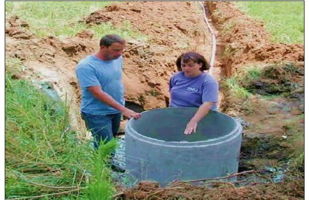
Springs are developed by removing obstructions to the flow and collecting the water. The type of collection system used for the spring development is dependent upon the type of spring and site geology. Collection systems generally consist of a restrictive barrier that forces water to collect in a perforated pipe that flows to an outlet.
