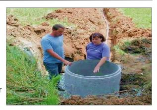
Springs are developed by removing obstructions to the flow and collecting the water. The type of collection system used for the spring development is dependent upon the type of spring and site geology. Collection systems generally consist of a restrictive barrier that forces water to collect in a perforated pipe that flows to an outlet.
