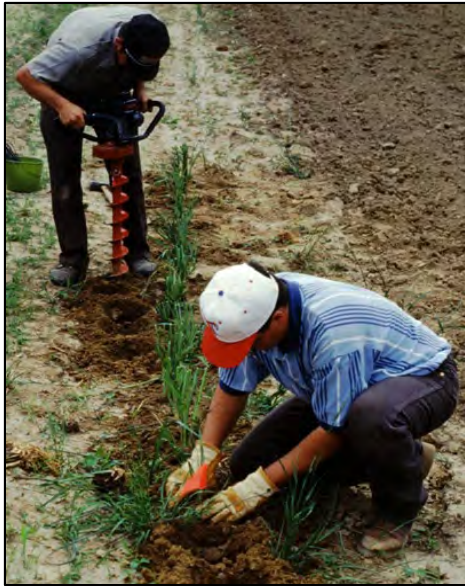
Figure 8: Repairing washout in concentrated flow areas using 'Alamo' switchgrass transplants.
