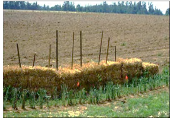
Figure 9: Haybales positioned across the concentrated flow area to protect new 'Alamo' switchgrass transplants.
