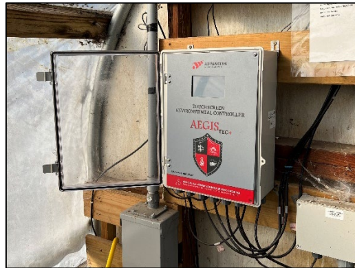
Typical environmental controller that raises and lowers the sidewalls based on temperature.
