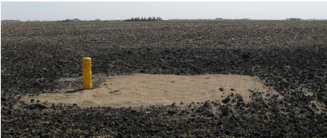
*Photo 1. Newly installed blind inlet in Hardin County, Iowa. The perforated riser was left in place for research purposes. (Photo by Martin Shipitalo, ARS-NLAE)*
