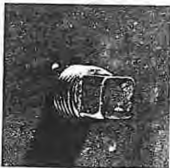
Figure 32. After completion of the test, remove the Collins tube and packing glands. Install 1/4" pipe plugs in the tapped hole. Tighten snugly.
