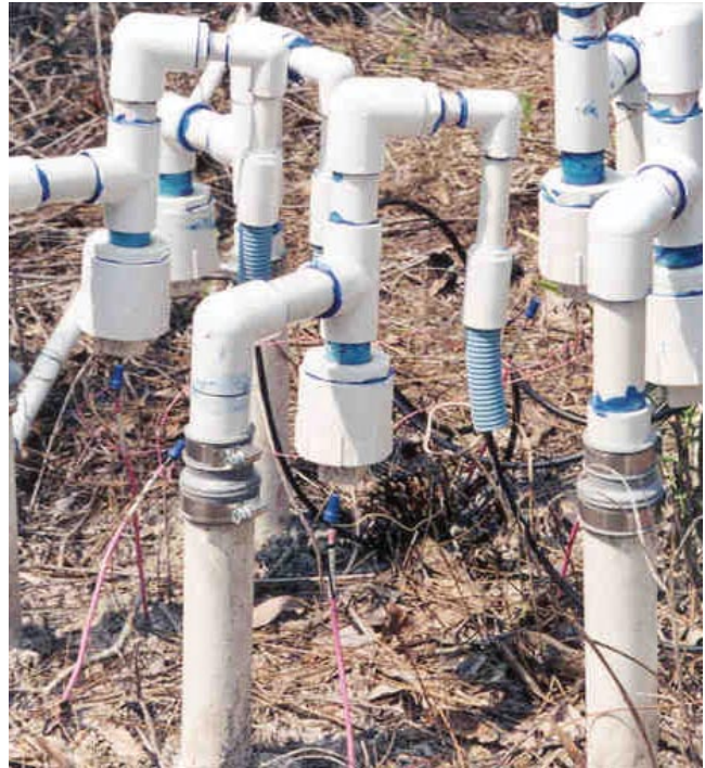
Figure 5.— Properly installed monitoring equipment (as described in the Hydric Soil Technical Standard) is important if one is to obtain approval of additions, deletions, or other changes to the hydric soil indicators.
