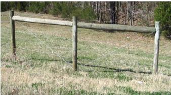
An H-brace is required for all barbed wire fences and electric fences with more than two wires. Since barbed wires fences need to be tight to be effective, a well-built H-brace is very important. This is in contrast to electric fence where the control is by animal fear of the electric fence and the fact that high tensile wire, especially single strand, should not be very tight.
