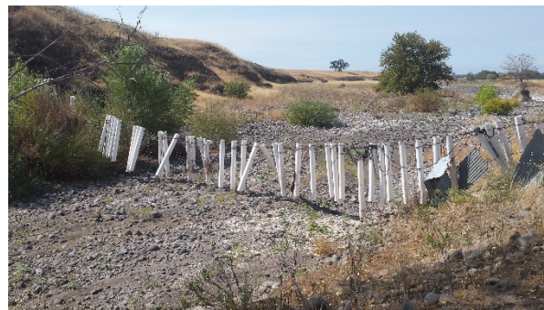
Deadman used for change in topography and a break-away fence crossing a draw
