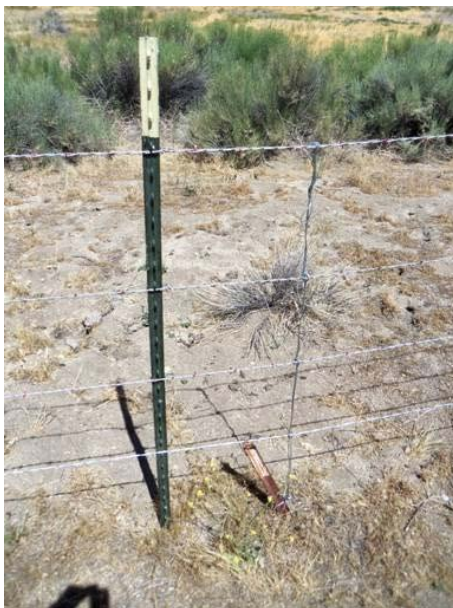
Deadman used for change in topography and a break-away fence crossing a draw
