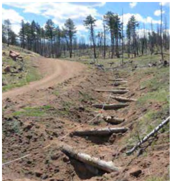
Figure 65: Log “rock and roll” channel in the Trail Creek watershed, Colorado (USFS 2015).
