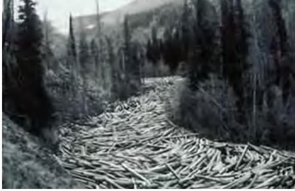
Figure 35: Railroad tie drives in the Rocky Mountains resulted in instream wood removal and reduction in channel variability (courtesy of the American Heritage Center).
