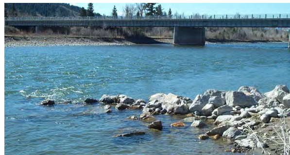
Figure 51: Stream barb (courtesy Jon Fripp).
