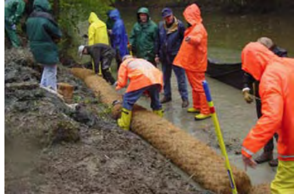
Figure 57: Installation of coir fascines (NRCS 2007, TS14I).
