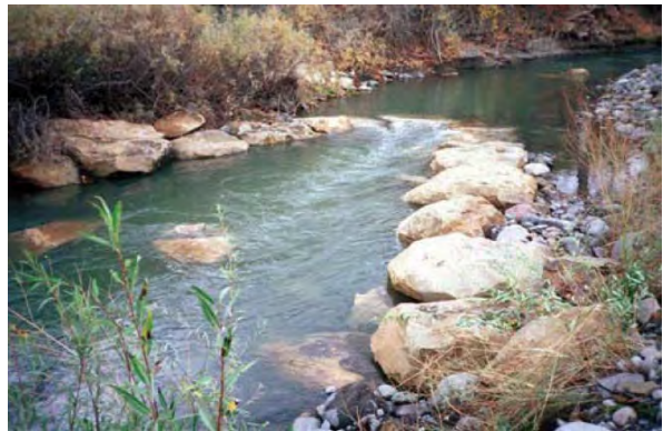
Figure 63: Cross vane on the Rio Blanco, CO (NRCS 2007, Ch11).
