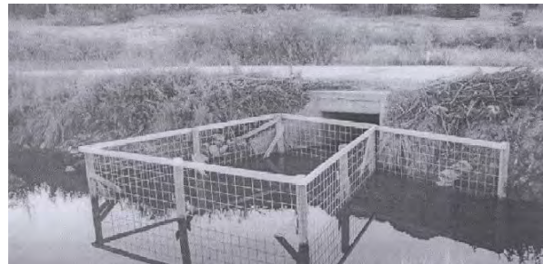
Figure 49: Beaver deceiver (Brown et al. 2001).
