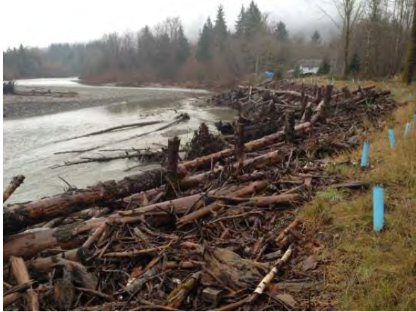
Figure 40: Complex timber revetment (photo credit: Tim Abbe, USBR and ERDC 2016).
