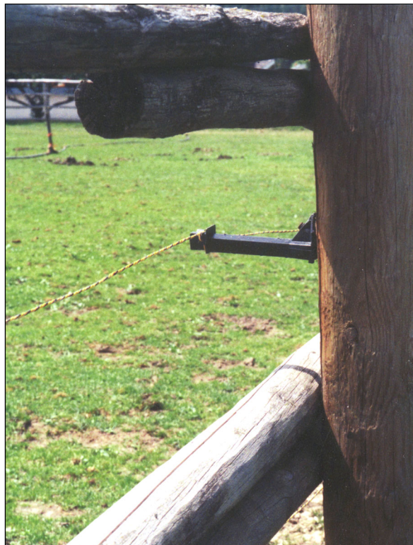
Figure 3 Typical Offset Line Post Insulator
