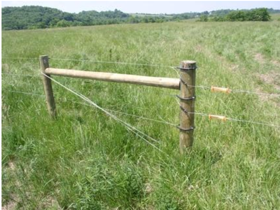
Figure 1. H-Brace End Assembly
