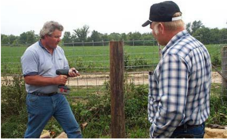
Drill hole to attach horizontal brace with pin
