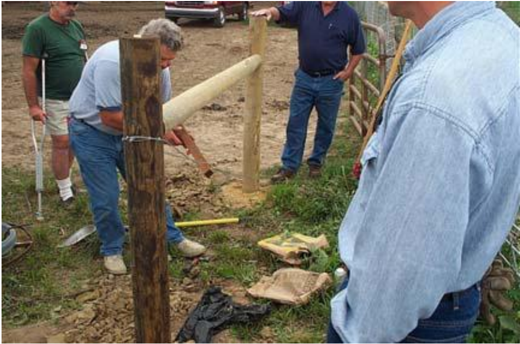
Attaching and tightening brace wire with twitch stick. Also may use ratchet tightener
