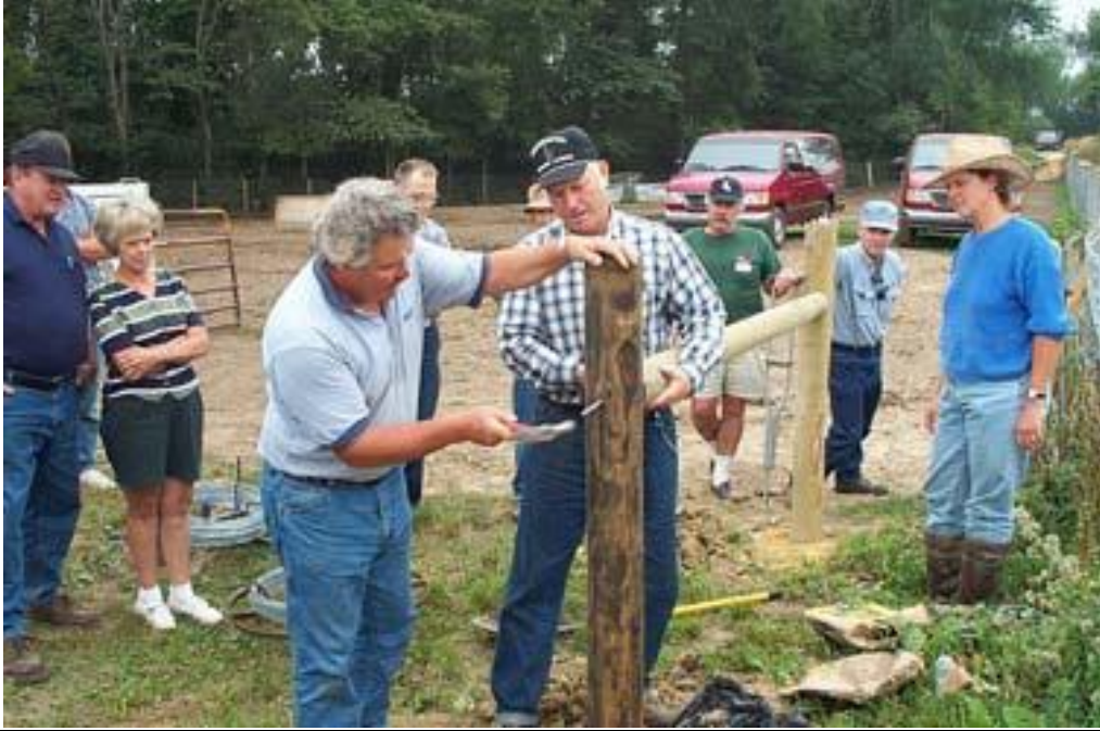
Attaching 10” Brace Pin
