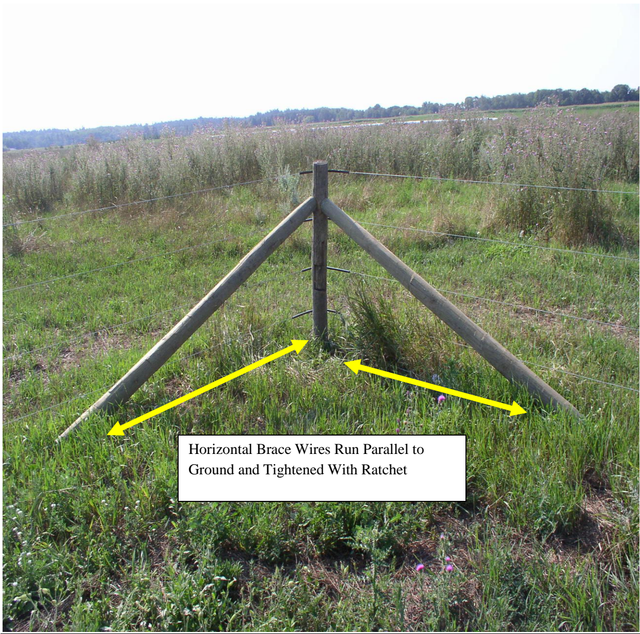
Figure 8. Double Floating Brace
