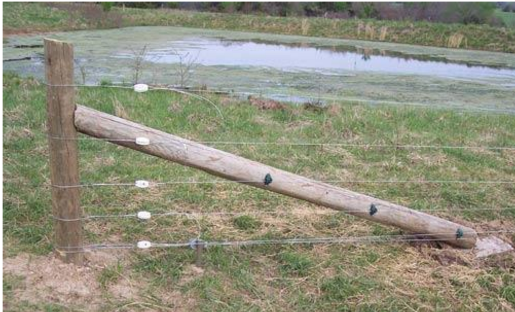
Figure 2. Floating Brace Assembly
