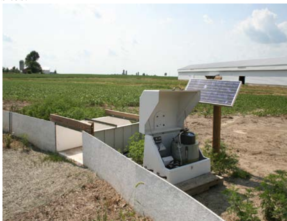
Figure 1: Edge-of-field surface runoff site with a 2.5 foot H-flume
