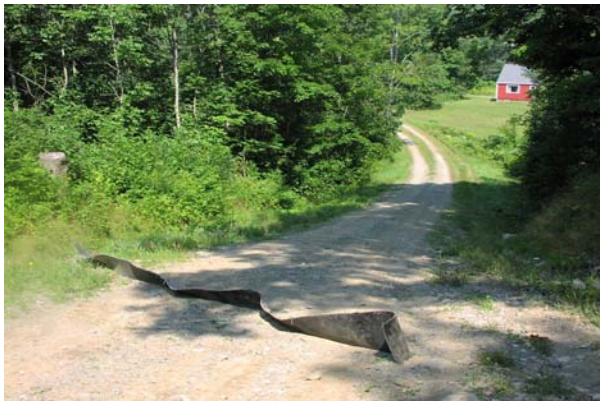
Machine belt erosion control on access road.
