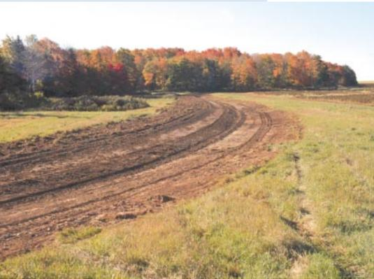
A diversion ditch was constructed to redirect runoff from crop land, direct it into sediment basins, and eventually into the deep pond.
