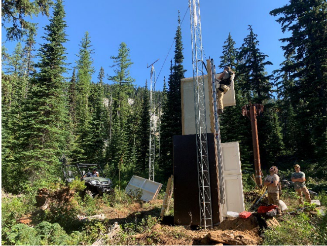
Left: Constructing a 16 foot shelter with the help of a winch. Right: Completed SNOTEL station at Chicago Ridge.
