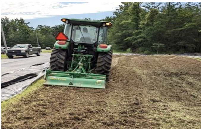
Figure 3.6. Rototilling a vegetated site to break up dense turf. Photo: NRCS/R Jay Ugiansky.
