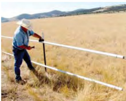
PVC pipe threaded over bunched fence wires creates an effective and durable big game passage.
