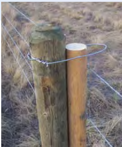
This lay-down fence using four-strand smooth wire was constructed along 1.5 miles of fencelines next to the Blackfoot-Clearwater Wildlife Management Area to allow winter passage for elk. The number of elk tracks attest to the design's success.
