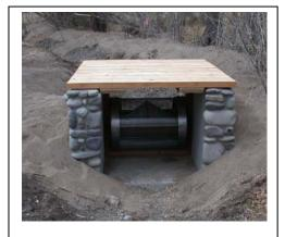
Screen set normal to channel with pipe bypass (not visible).
