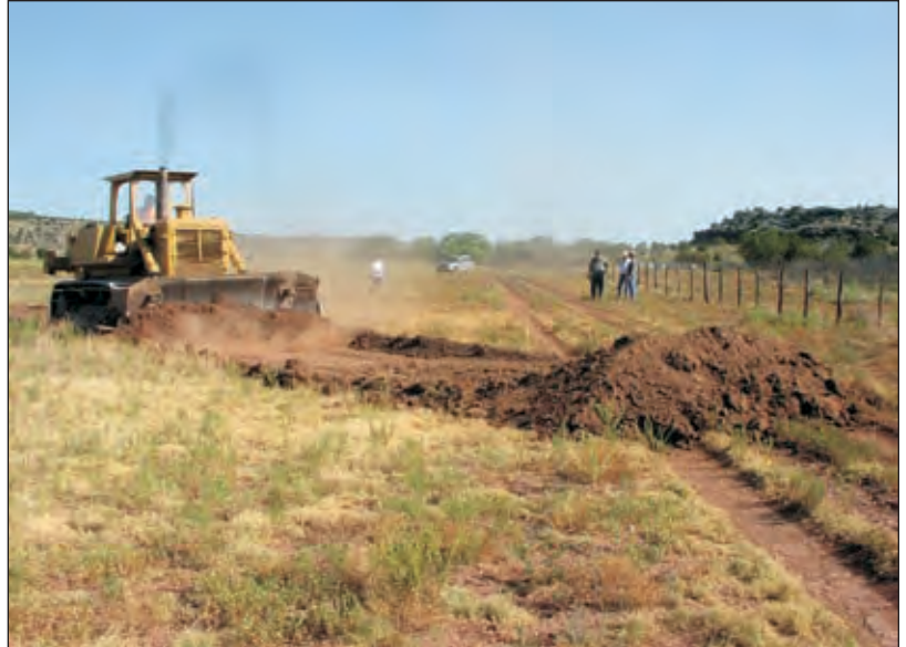
Photo V-9: Material borrowed from lead-out ditch is stockpiled on roadway.
