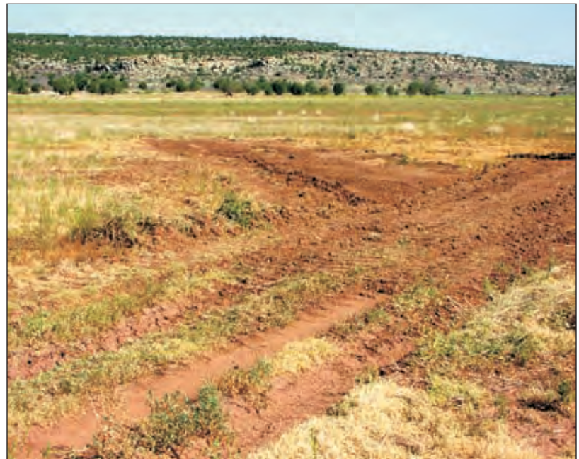
Photo V-11: Completed flat land drain and lead-out ditch on fine-textured soil. If needed, harden the surface with gravel hauled from another source.
