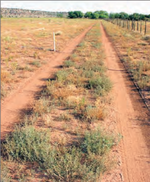
Photo V-8: A flat road on flat land. The stake marks the location of the planned drainage outlet.
