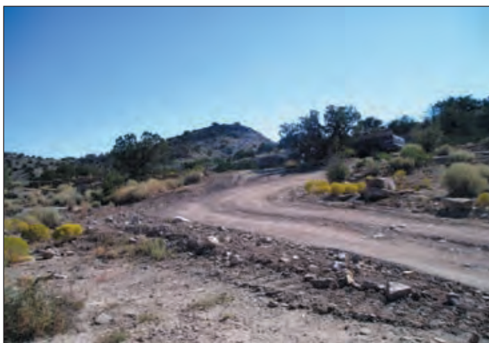
Photo V-2: An outsloped road with coarse-textured surfacing and berm removal.
