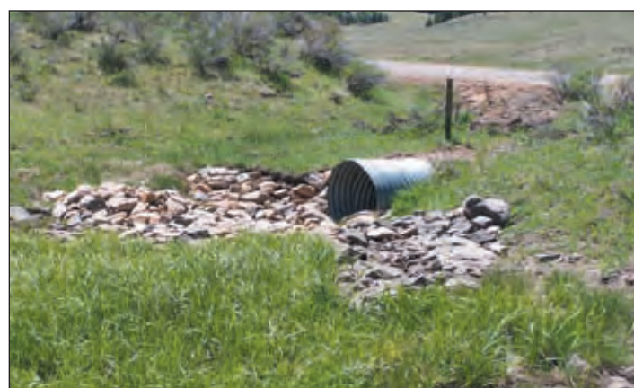
Photo VIII-5: A raised culvert inlet with recovering wet meadow vegetation.
