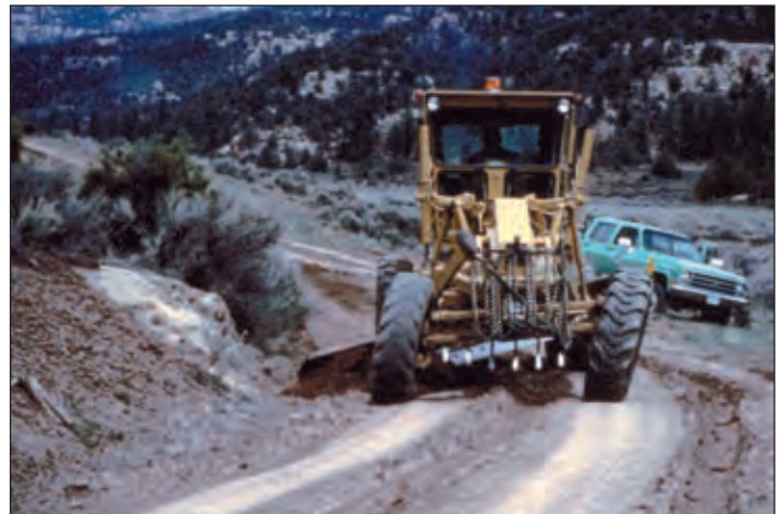
Photo V-3: Blading to maintain an insloped road template.
