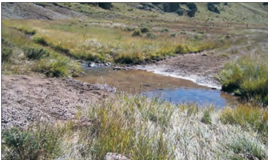
Photo VIII-1: Unimproved fords are commonly used stream crossings on low standard roads. A road should cross at right angles to the direction of the flow to avoid stream capture.
