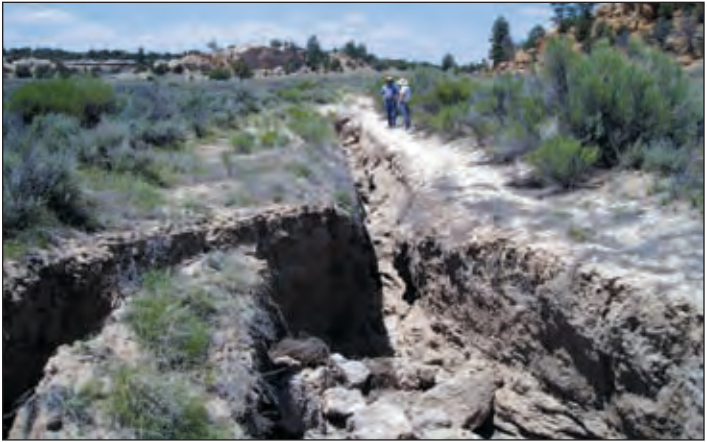
Photo I-3: Soil erosion resulting from concentrated runoff from an unpaved rural road.
