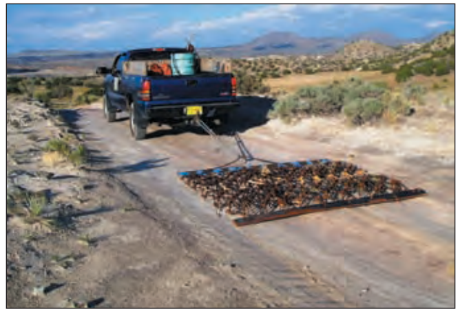
Photo IX-9: Chain harrow pulled behind a pickup to smooth the road surface. Such harrows can also be used to scarify the roadside for seeding.
