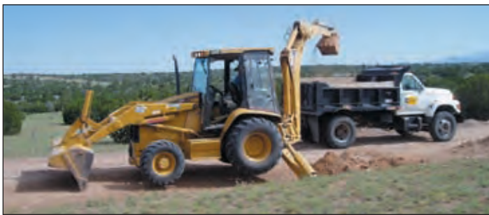
Photo IX-2: Backhoe removing sediment from a culvert inlet.
