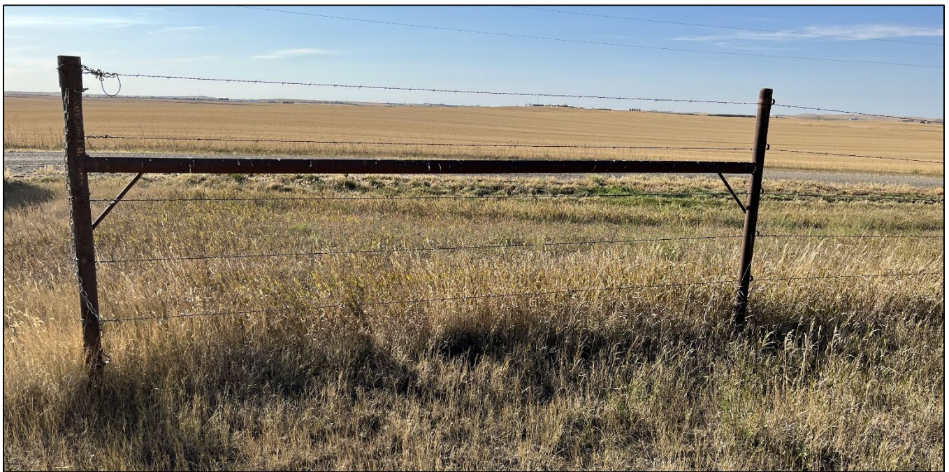
Photo 6. All steel H-brace. Photo by USDA-NRCS.
