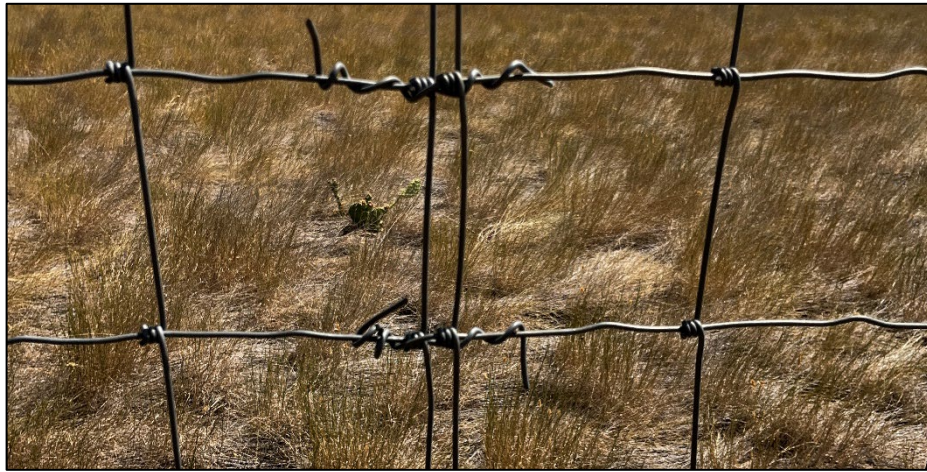
Photo 3. Close-up of fence splice on woven wire fence. Photo by USDA NRCS.
