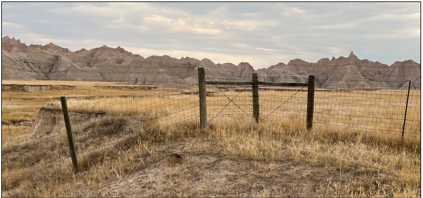
Photo 5. Woven wire bison fence with H-braces installed at corner change. Photo by USDA-NRCS.
