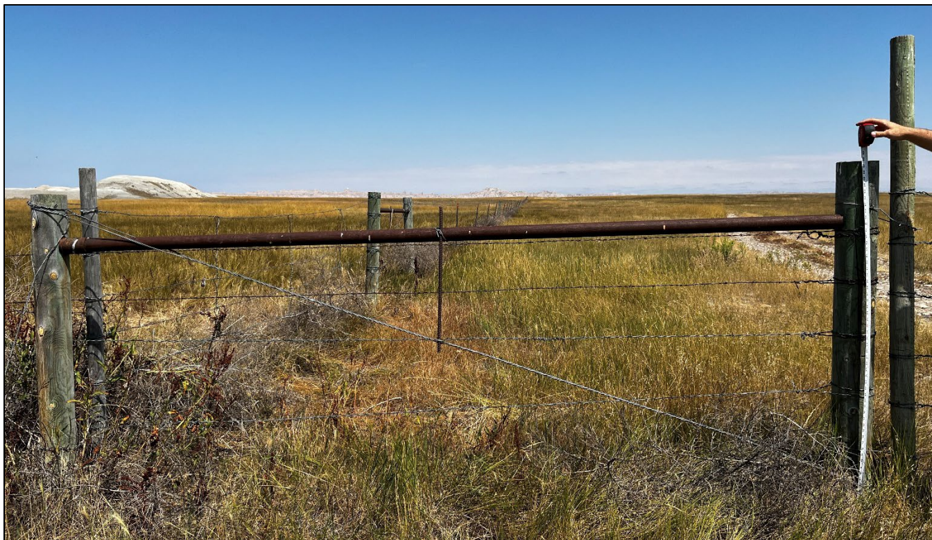
Photo 1. Bison fence gate brace. Photo by USDA NRCS.
