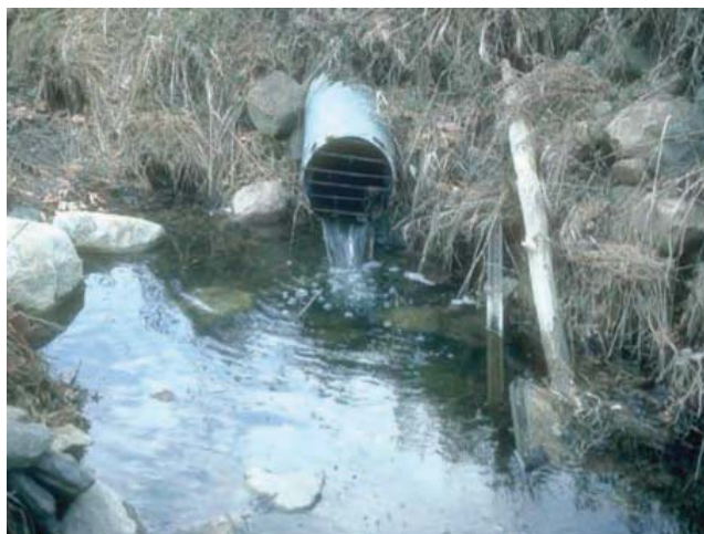
Figure 17.19. Subsurface drain line discharges into an edge-of-field ditch, diverting groundwater to surface waters.
