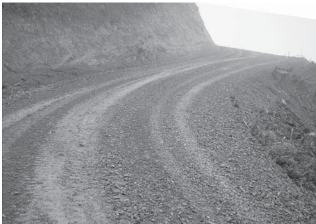
Figure 3-1. A full bench outsloped road section on a 70% slope.
