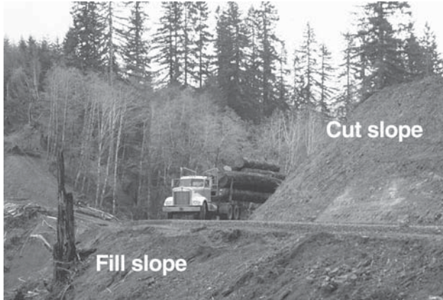
Figure 1-8. Example road cut and fill slope.
