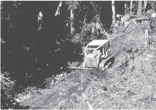
Figure 4-6. Tractor constructing road subgrade.
