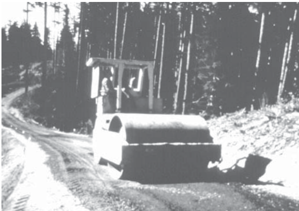
Figure 4-15. Smooth-wheel vibratory roller compacting surface rock.
