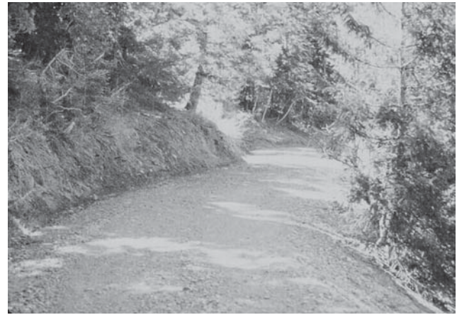
Figure 4-9. Road constructed with well-compacted and -drained subgrade.
