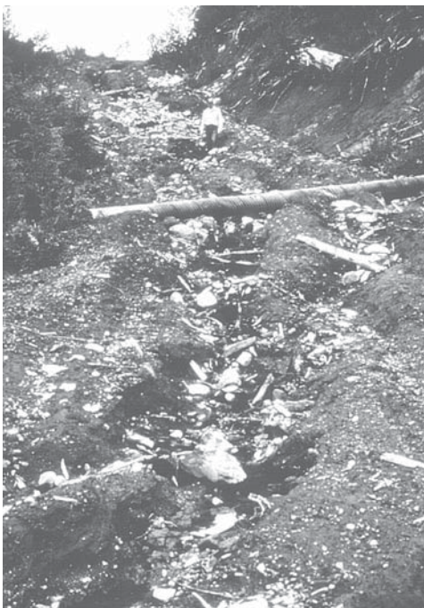
Figure 6-10. Catastrophic ditch and roadway erosion.
